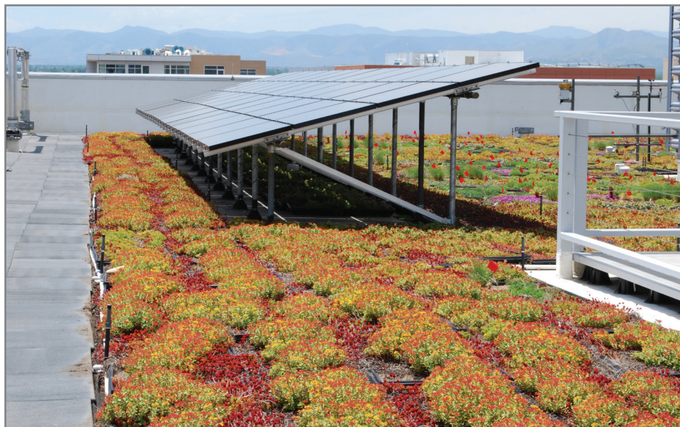
Tom Slabe, Green Roofs of Colorado The U.S. Environmental Protection Agency Region 8 headquarters' rooftop in Denver
